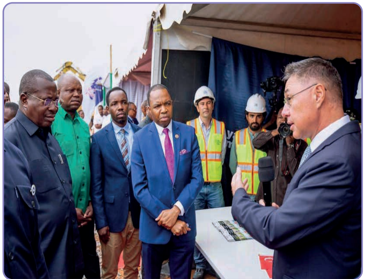
Vice President Dr Philip Mpango listens as Yapi Merkezi deputy manager explains about the Tabora-Isaka SGR railway section works, at Isaka, Shinyanga, January 18, 2023
